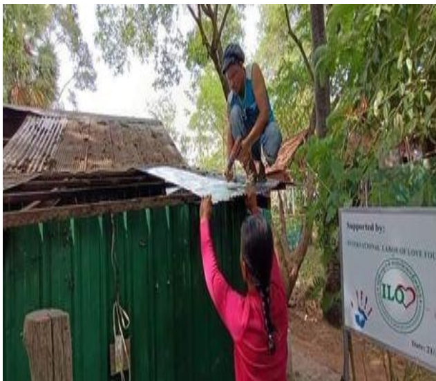
SCC-SBE staff removed the old zinc of the roof in the kitchen building instead the new one on June 2021
